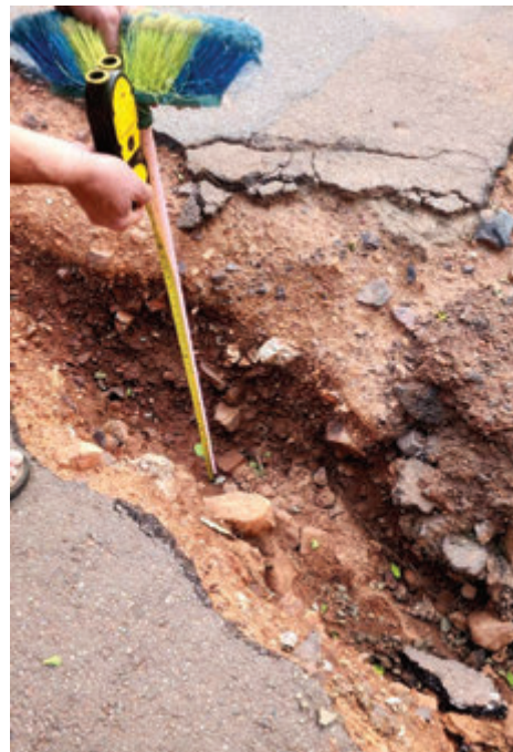
Residents measured the depth of a massive pothole at the Bokmakierie/ Hamerkop intersection in early 2026. Although Thabazimbi Local Municipality later filled the hole, it was reportedly patched with sand and has since begun forming again — raising concerns about the lack of a long-term solution.
